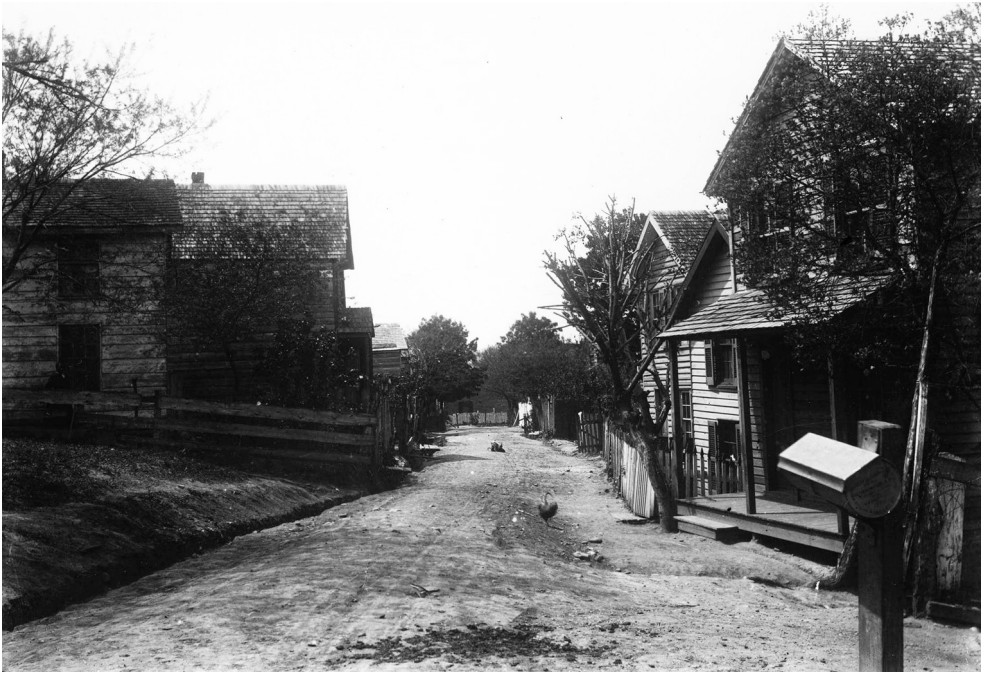
Figure 7. This 1910 photo of East Arlington shows unpaved streets, no gutters, no sidewalks. By 1942 when it was leveled to make way for the Pentagon, Arlington County had still not run water or sewer to East Arlington. Photo reproduced with permission of the Virginia Room, Arlington Public Library.
