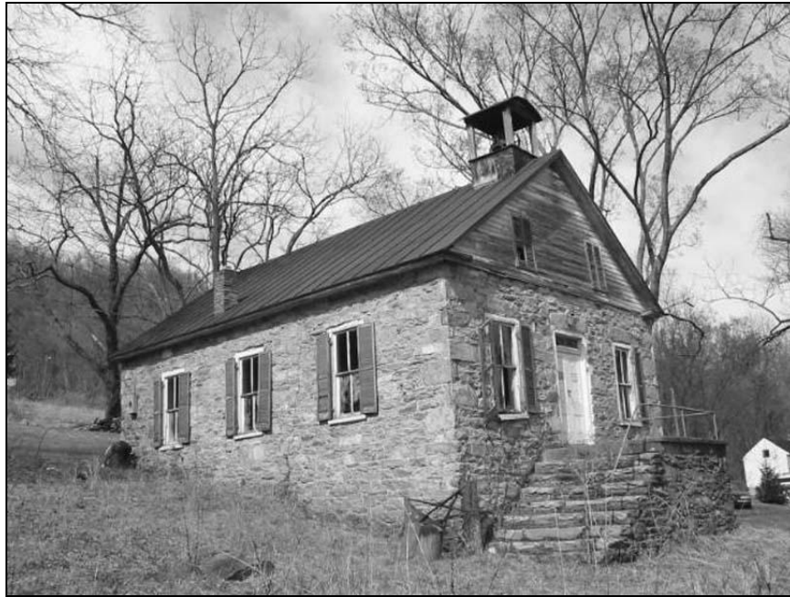
Figure 27. Asbury Methodist Episcopal Church, Hillsboro vicinity. South and east elevations (DHR #053-0909).
