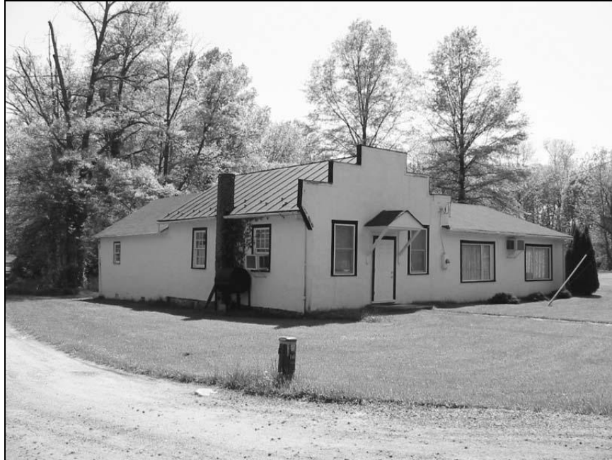
Figure 13. Store, 35285 Snake Hill Road, St. Louis. South and west elevations (DHR #053-5099-0009).
