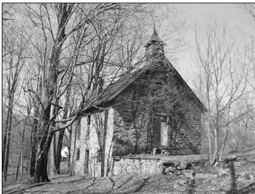
Figure 26. Grace Methodist Episcopal Church, Lincoln. South and east elevations (DHR #053-0205).
