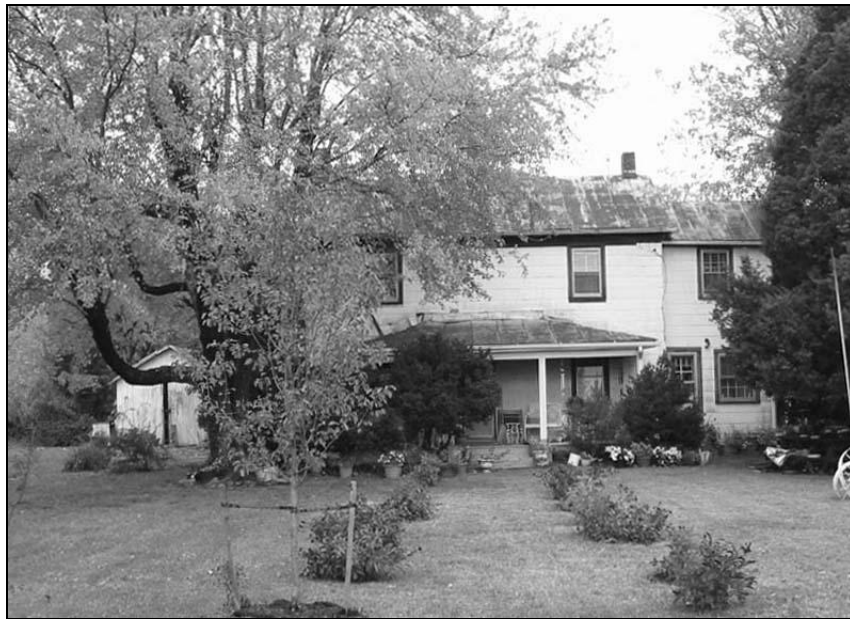
Figure 28. Nokes House, Nokesville. Façade or south elevation (DHR #053-5223).
