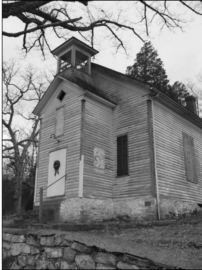
Figure 25. Mount Pleasant Baptist Church, Bowmantown. Façade or east elevation (DHR #053-1023).
