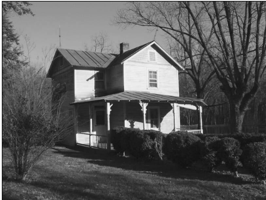
Figure 19. House, 24060 New Mountain Road, Bowmantown. North and west elevations (DHR #053-0605-0007).
