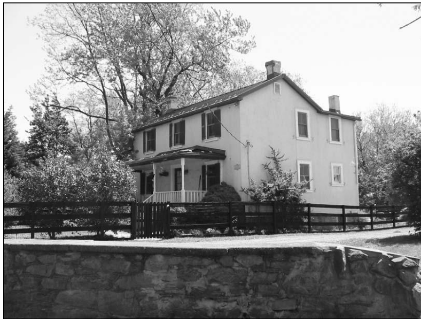
Figure 15. Brown Family House, Macsville. North and west elevations (DHR #053-5151).
